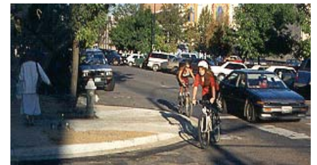
Horizontal —Bulb-out at an intersection
