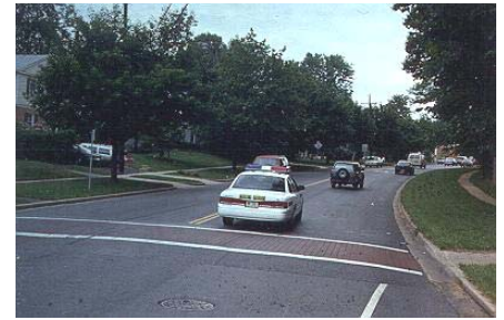
Passive —Use of contrasting materials to clearly define crosswalks
