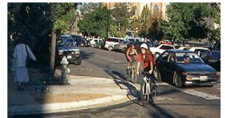
Horizontal —Bulb-out at an intersection
