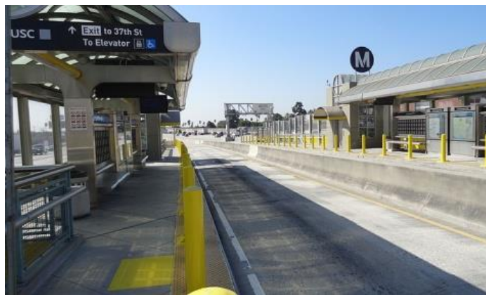
Figure 5-2: In-Line Station on I-110
