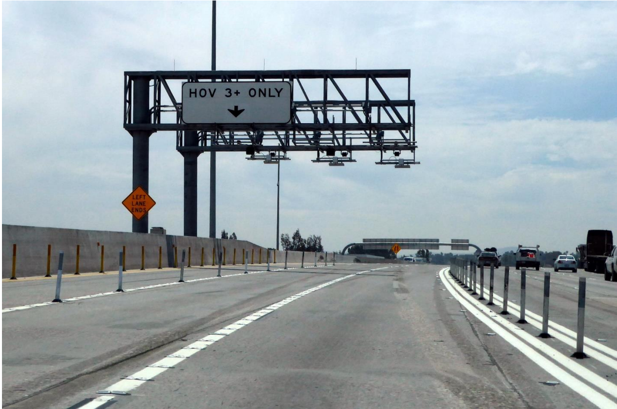
Figure 4-2: Sample Channelizer Separation with HOV Declaration Zone, SR-91 Express Lanes, Riverside, California
