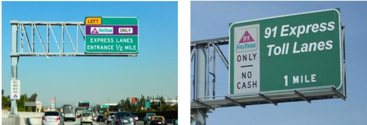
Figure 4-8: Express Lane Entrance Signage
