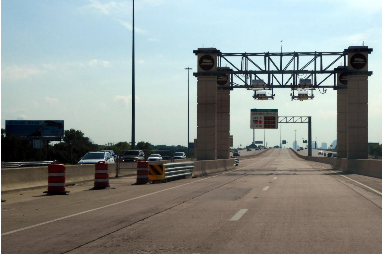
Figure 4-5: Sample Barrier Separation, I-30 Express Lanes, Dallas, Texas
