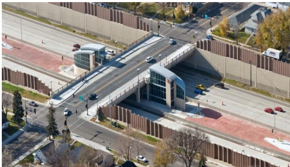
Figure 4-12: In-line BRT station on I-35W Express Lanes, Minneapolis, Minnesota
