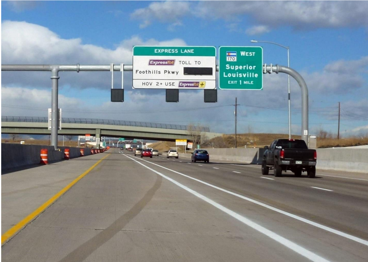
Figure 4-3: Sample Buffer Separation, U.S. 36 Express Lanes, Denver, Colorado.
