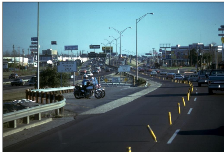
Figure 4-11: I-45 Enforcement Area, Houston
