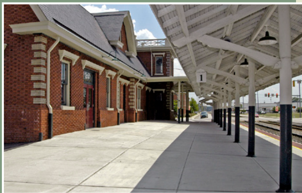
Built in 1911, the Fayetteville Train Station serves four trains daily.
