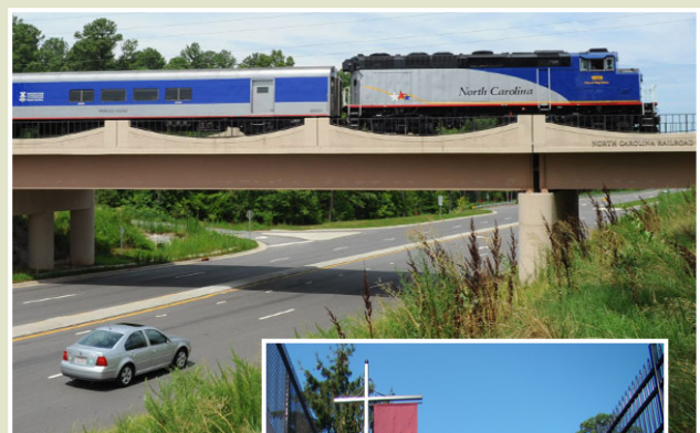
NCRR Bridge over NC 54
