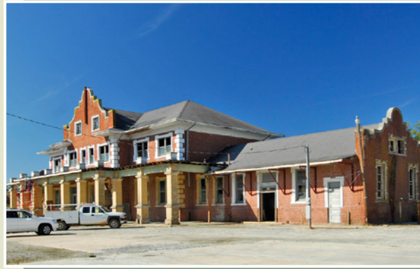
Goldsboro Union Station was stabilized for future use.
