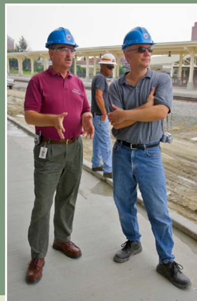
Allan Paul, left and Craig Newton on construction site at Greensboro Depot
