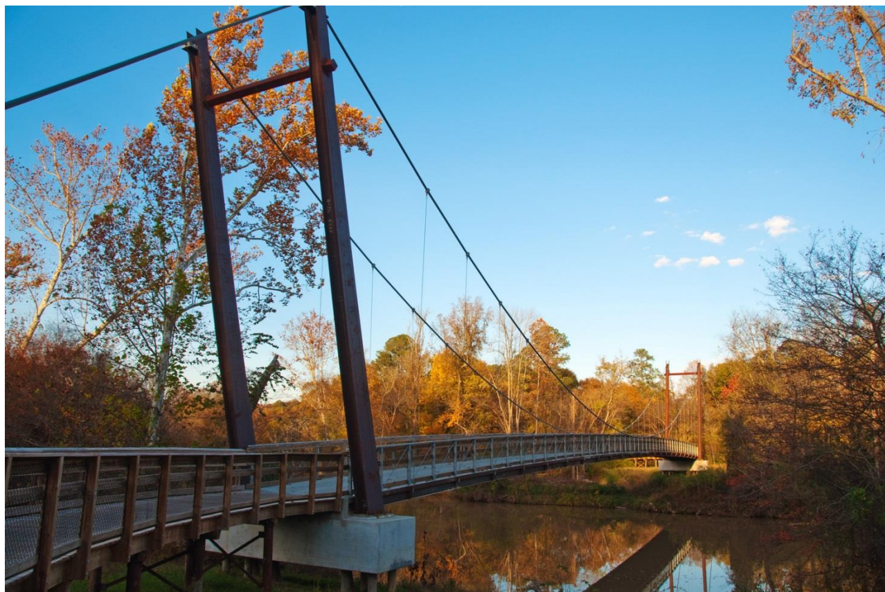
Figure 1: Example of Aesthetics--Neuse River Greenway Bridge. [Image By Bz3rk - Own work, CC BY-SA 3.0, https://commons.wikimedia.org/w/index.php?curid=29878720 ]
