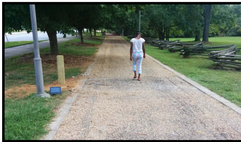
Figure 1. Continuous Count Station Installation
