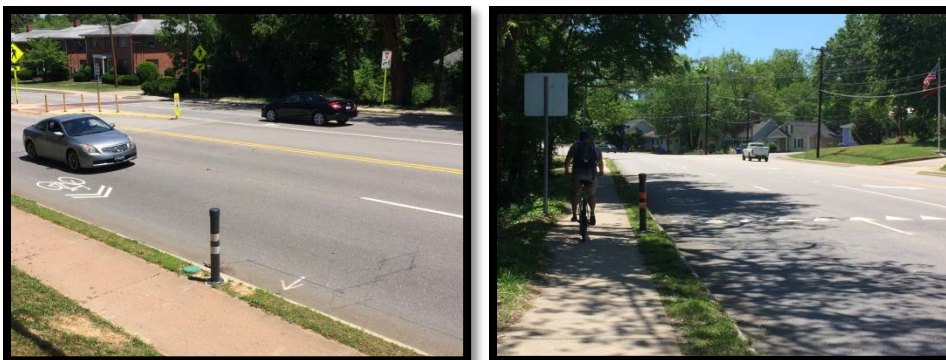
Figure 1. Continuous Count Station Installation West (Left) and East (Right)
