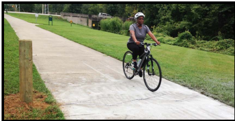
Figure 1. Continuous Count Station Installation
