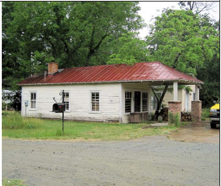
Site # 4: Former Gas Station. View to the northeast.
