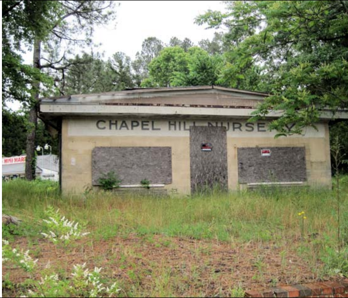
Site #1: Former Chapel Hill Nursery. View to the east.
